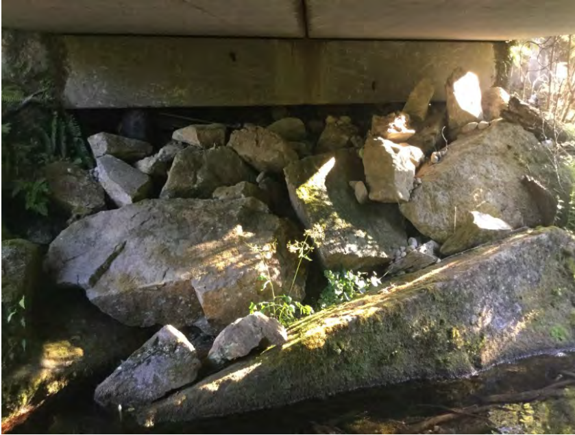
Left Bank Abutment
