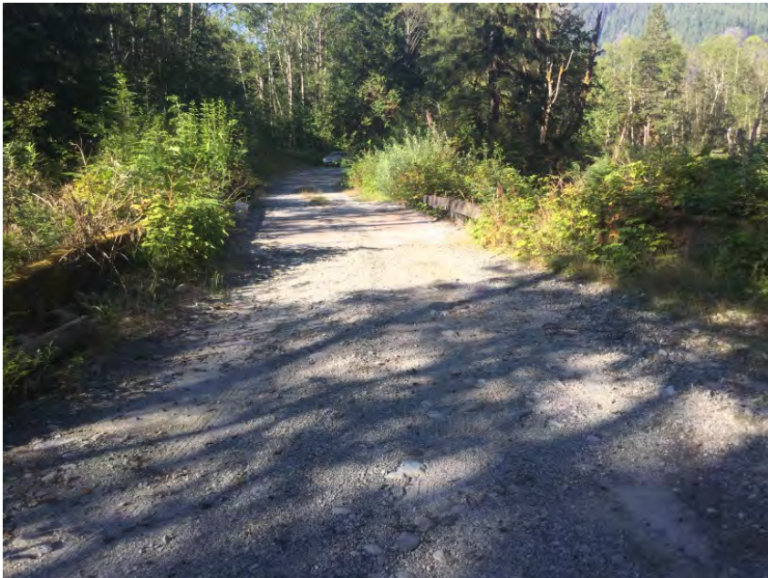
Left Approach Facing Bridge
