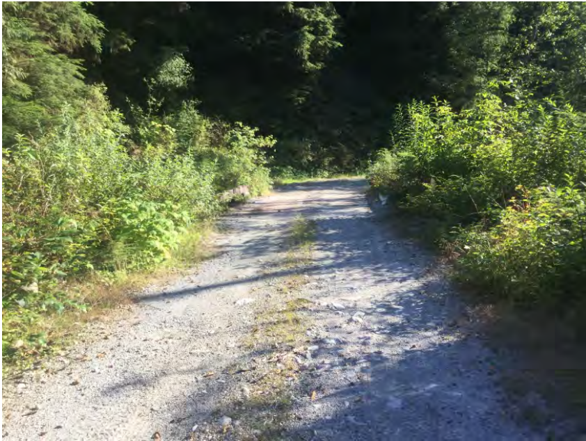
Right Approach Facing Bridge
