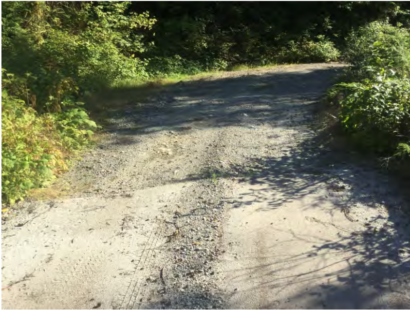
Left Approach Facing Away From Bridge
