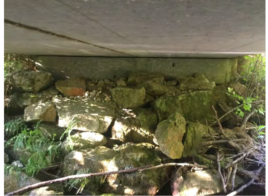
Right Bank Abutment
